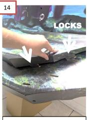
Close-up view of the lock tabs on the **SIGN BASE.** Make sure all sides are overlapping correctly so the locks will engage easily.
